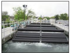
The new facility, which can handle up to 800,000 gallons a day, with future expansion to 1.2 million gallons, will be large enough to allow extension of the sewer system to East Patchogue.
